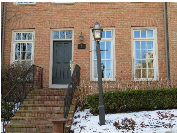
Light pole lean, shown at Unit 5
