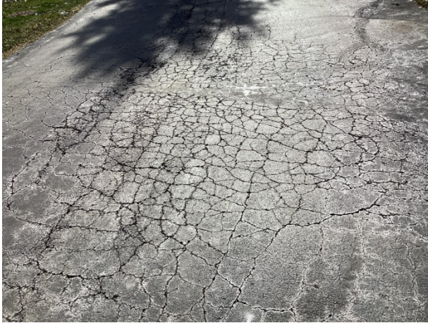
Alligator cracks
