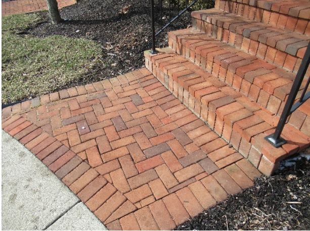
Brick stairs overview
