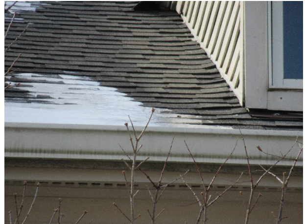
Shingle lift, shown at Unit 2
