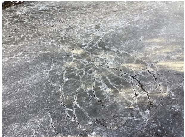
Alligator cracks
