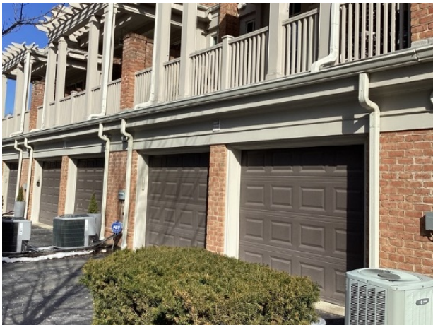
Gutters and downspouts overview
