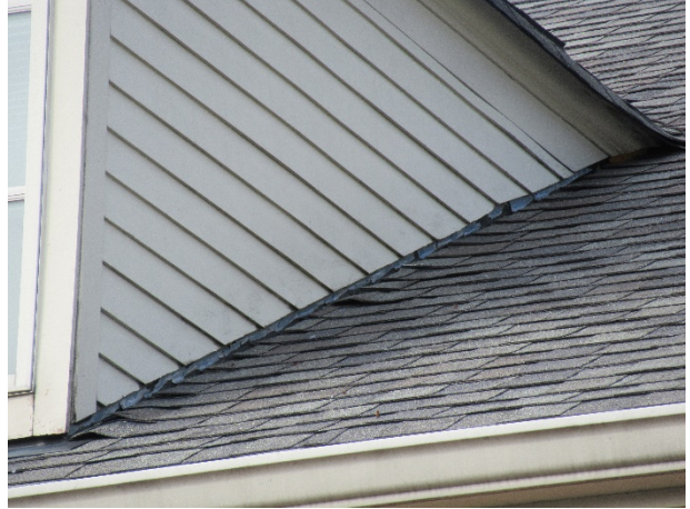
Shingle lift, shown at Unit 7
