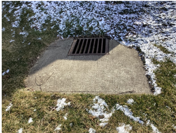
Landscape catch basin
