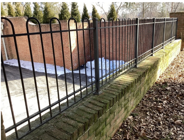
Railing at retaining wall
