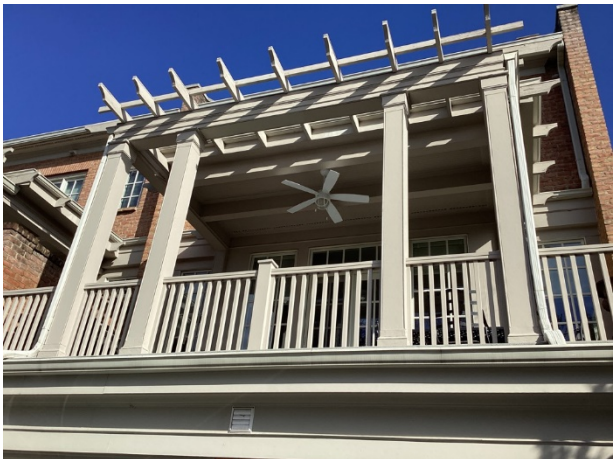
Pergola and railings overview
