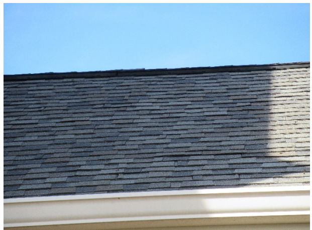
Shingle lift, shown at Unit 13
