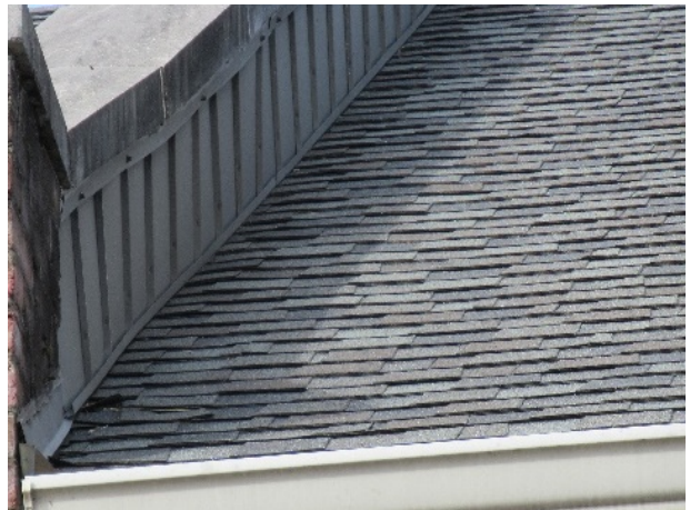
Shingle lift, shown at Unit 9
