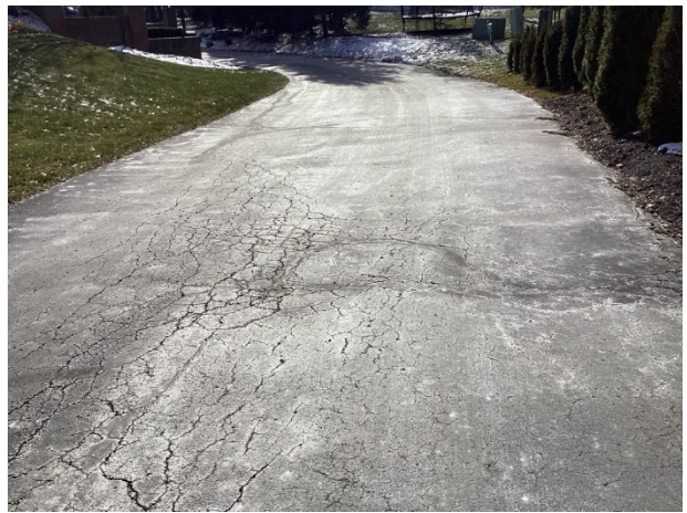
Access drive overview
