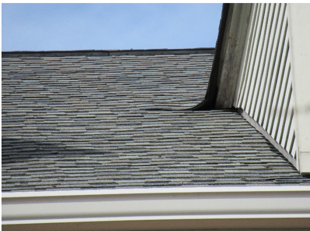
Shingle lift, shown at Unit 12
