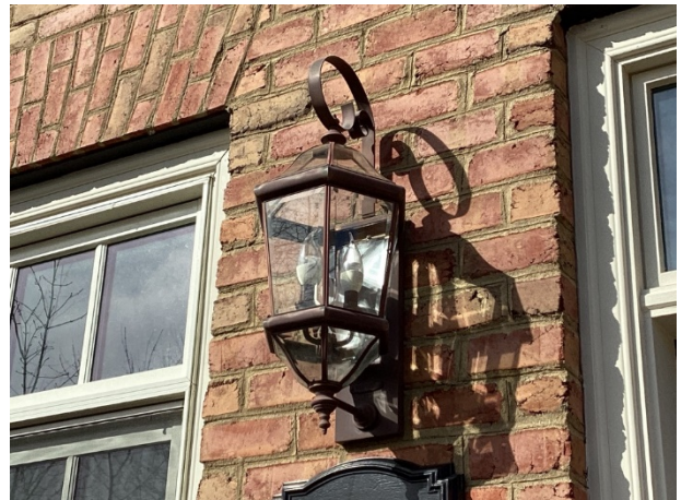
Light fixture at Units 10-13
